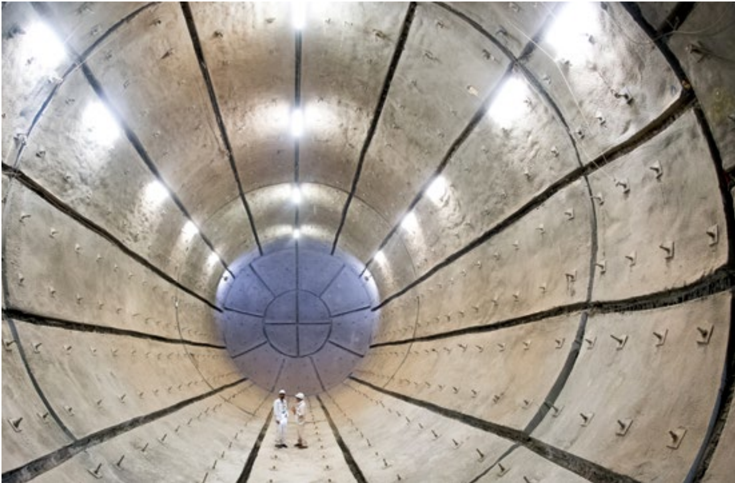
At Your Disposal Two men stand in the Konrad shaft nuclear repository being built in an abandoned iron ore mine in the city of Salzgitter in Germany. The deep mine will store low- and medium-level radioactive waste. As Richard Ovenden reminds us, “As a society we really need to be sure we will know long into the future ... exactly where we have stored nuclear waste, what material it consists of, when it was placed there, what kind of container it was stored in, and so forth.... Sound familiar? It’s called good archival practice.” PHOTO: JULIAN STRATENSCHULTE/PICTURE ALLIANCE VIA GETTY IMAGES
